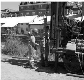
Boreholes were drilled to determine the character of the soil on each side of the dock. This is being done to ensure the ship in the dock dry for a protracted period of time and visitors will be safe.
