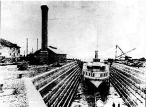
The keel of the ship has to pass over the sill of the dry dock with only inches to spare. There one chance to do this and that is during a few critical weeks of high water in June each year. The dry dock is an industrial monument and has designated a National Historic Site. This photo shows the drydock as it was in 1891, with the sidewheel steamer *St Lawrence*, the first vessel to use the drydock.
