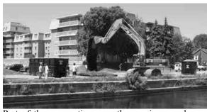
Part of the preparation over the previous week was putting gravel filled dumpsters in place to take the ships lines. The strength of the existing dock bollards is yet to be tested.
