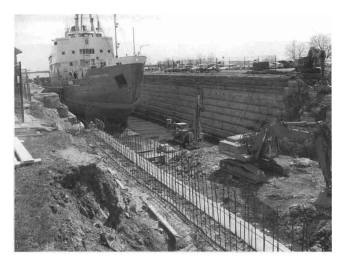
April 2010. The new east wall is now well advanced and can be seen on the left foreground. On the right (and just out of sight) the Doomekamp Construction crew are laying the foundation for the new west wall. The 1890 limestone steps have been cleaned and silt is being removed from the bottom of the dock.
