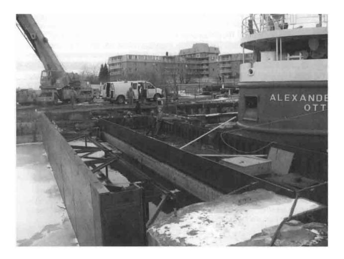
**February 2010.** There are two dry dock caisson positions. Normally the inner position is used, but should extra length be needed for a docked ship, the caisson can be shifted to the outside position. On the left the new cofferdam, built for this project is in the outside or seaward position. The original 1890 Caisson is preserved in the usual position immediately aft of the Museum Ship *Alexander Henry*.
