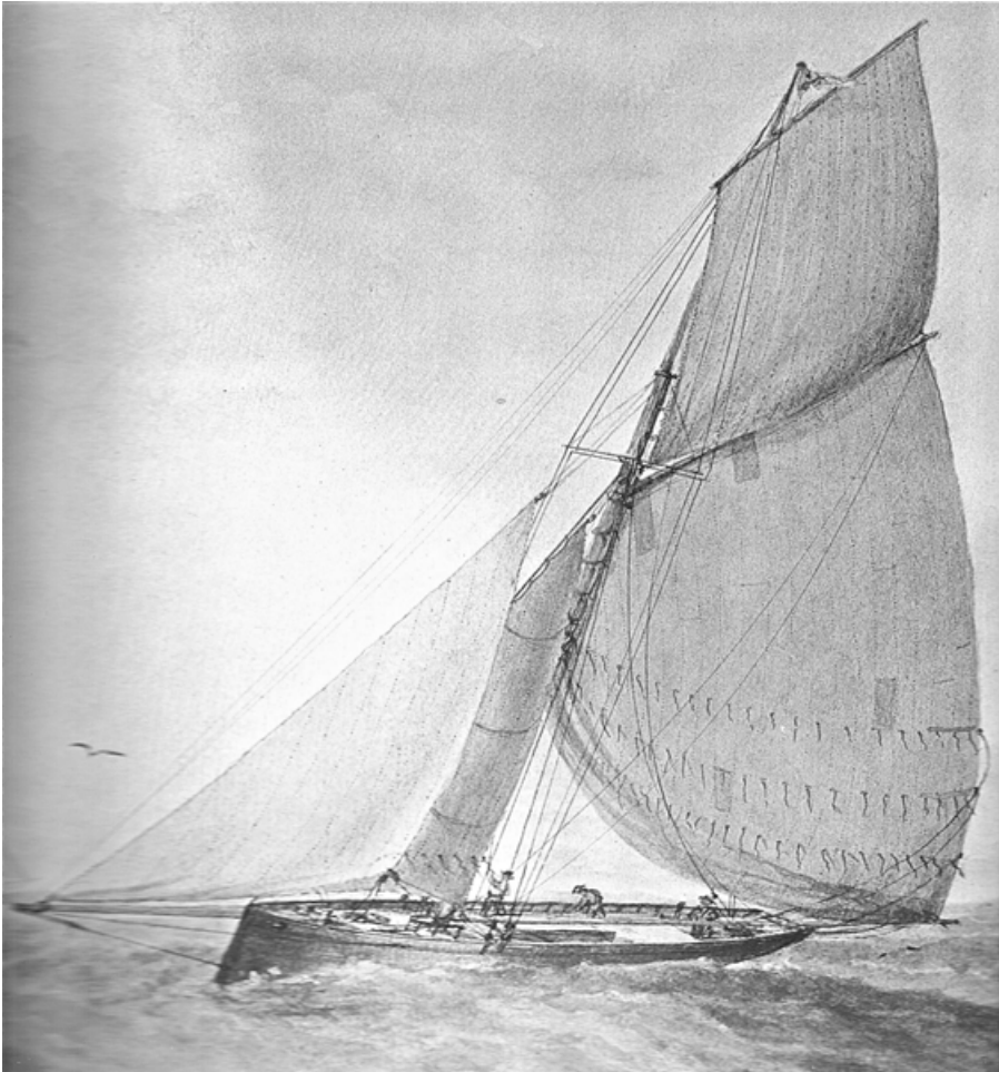
(Figure 2) Verve I in the process of gybing. Raising the tack was one way of “de- powering” the mainsail. Note the blunt bow. William Armstrong painting. [Campbell. Early Days on the Great Lakes ]
