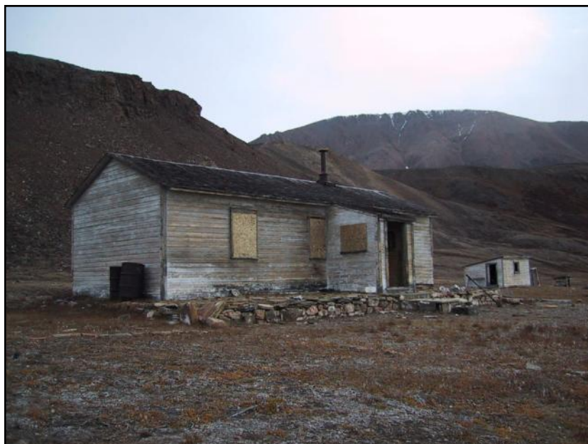
Deserted RCMP building, Dundas Harbour ( D.Riedel, 2007)
