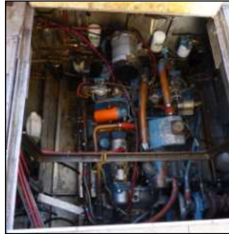
Engine Compartment Photo Source: Author
