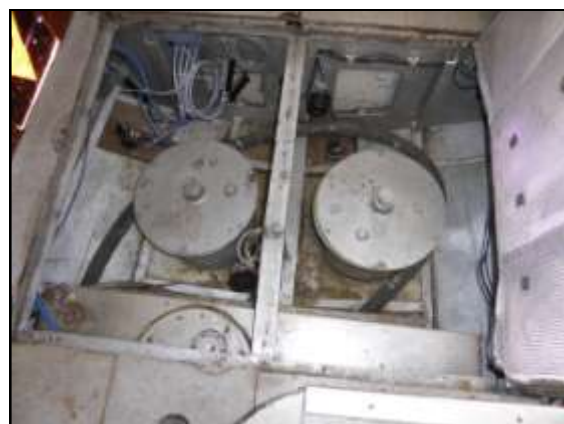
Port and Starboard Sonar Wells Photo Source: Author
