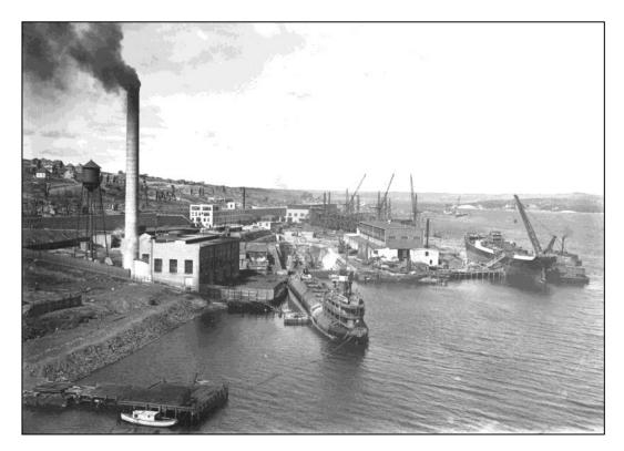
The Halifax Shipyard in 1920, having been rebuilt after the Explosion. Submarines *CH-14* and *CH-15* are shown in the Graving Dock, SS *Canadian Mariner* is alongside the Machine Shop wharf, and the whaleback barge *Atikokan* is in the foreground. The new building slips can be seen just behind the Machine Shop.
