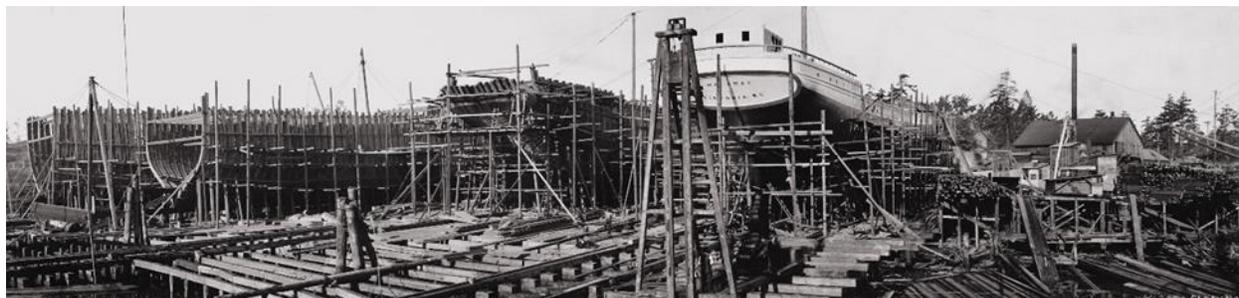
**Image 3:** *Malahat* building on Cameron-Genoa Mills Shipbuilding ways, 1917. What is probably the *Jean Steedman* and two of four wood cargo steamers also built by the company in the midst of construction lie off to the left. Photo courtesy of Ronald Greene, Capital Iron collection, Victoria.
