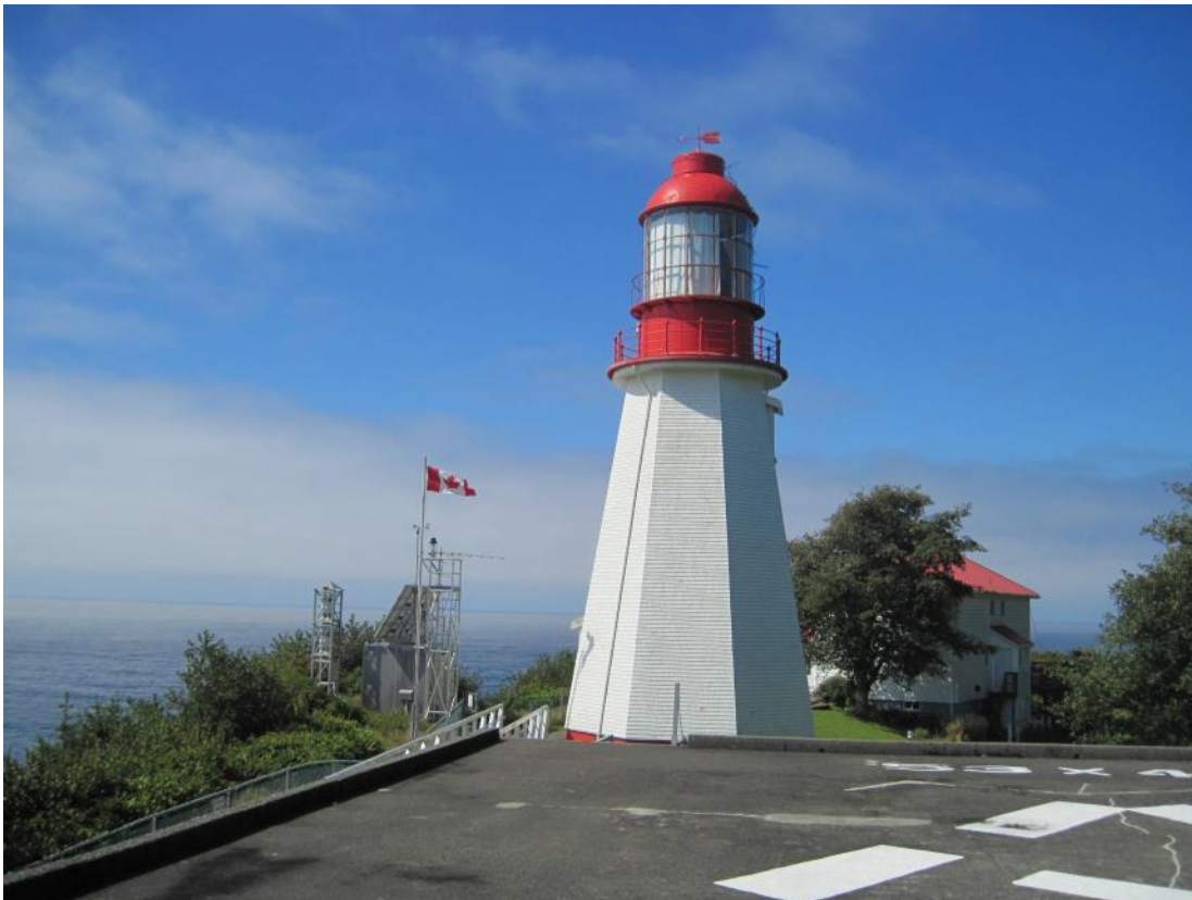
Figure 1: Looking out from the helicopter landing pad across the Pacific past Pachena Point light tower, the only remaining wooden lighthouse along our West Coast, completed in 1908 and recognized under the Heritage Lighthouse Protection Act . Its priceless and massive Fresnel lens, which revolved in a bath of mercury to produce a double flash every 7.44 seconds, is still there up in the tower and behind curtains in the lantern room. Photo Rick James.
