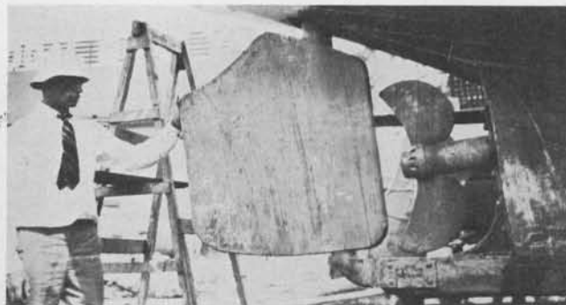
Reversible propeller with blades turned fore and aft for sailing.
